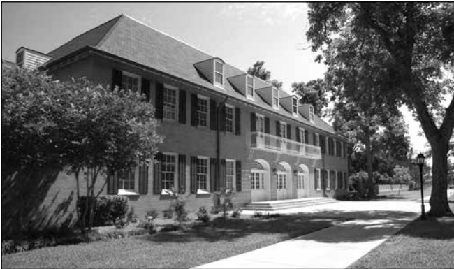
M.E. Dodd Building
